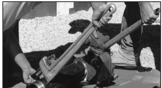
Figure 3: Attach Riser
