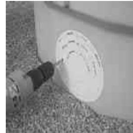
3. Use a hole saw to drill out the pipe entry hole.
