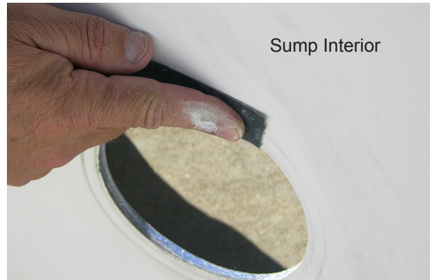
Figure 9: Sand Around Hole Interior
