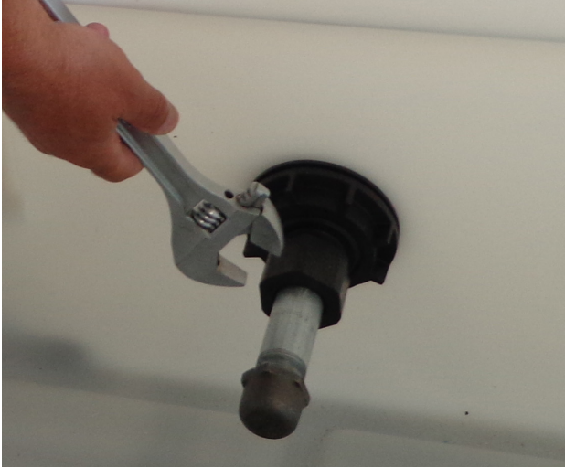
Figure 7: Insert Conduit and Tighten Compression Nut
