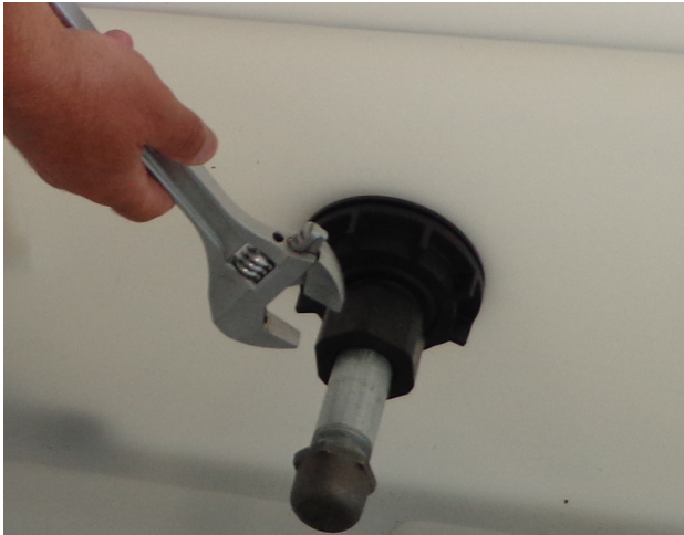
Figure 16: Insert Conduit and Tighten Compression Nut
