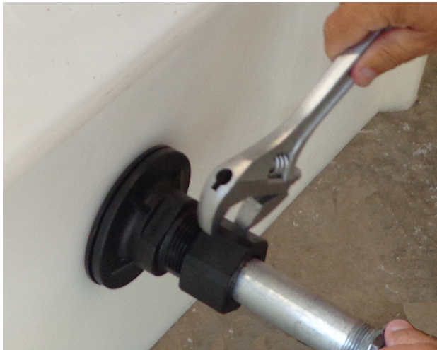
Figure 8: Tighten Outside Compression Nut
