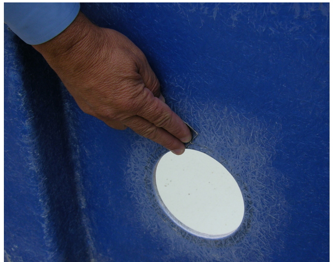
Figure 10: Sand Around Hole Exterior
