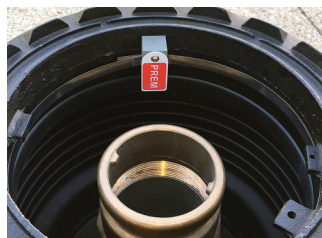
UST RFID tag mounting bracket XD281
