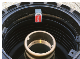
UST RFID tag mounting bracket XD281
