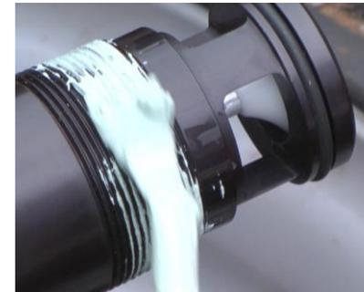
Figure 11-3 Apply Thread Sealant
