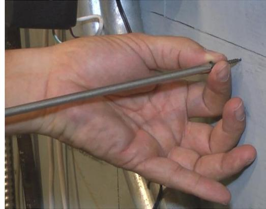
Figure 3-1 Install Hanger Screws
